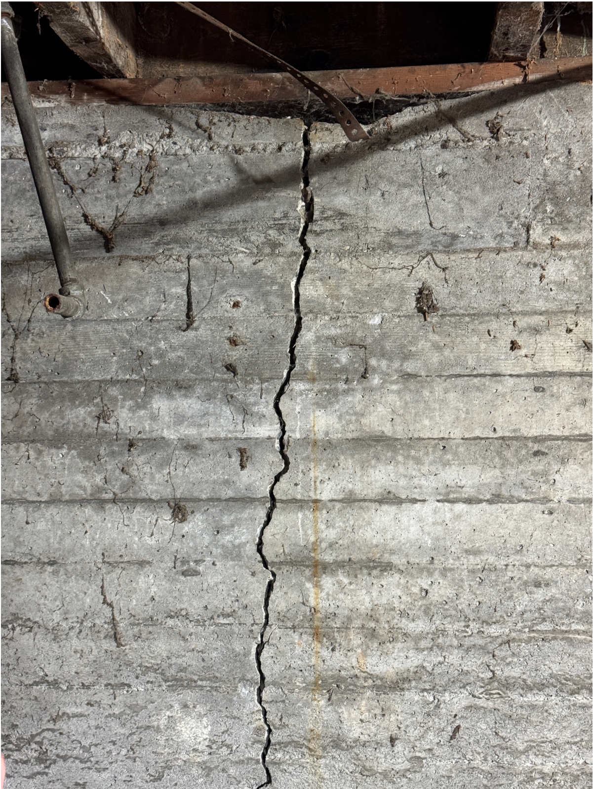
Foundation crack
